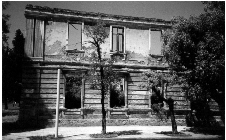
Destroyed building in Sukhum(i) PHOTO: ANNA MATVEEVA
