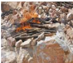
Firewood being used to break stones.
